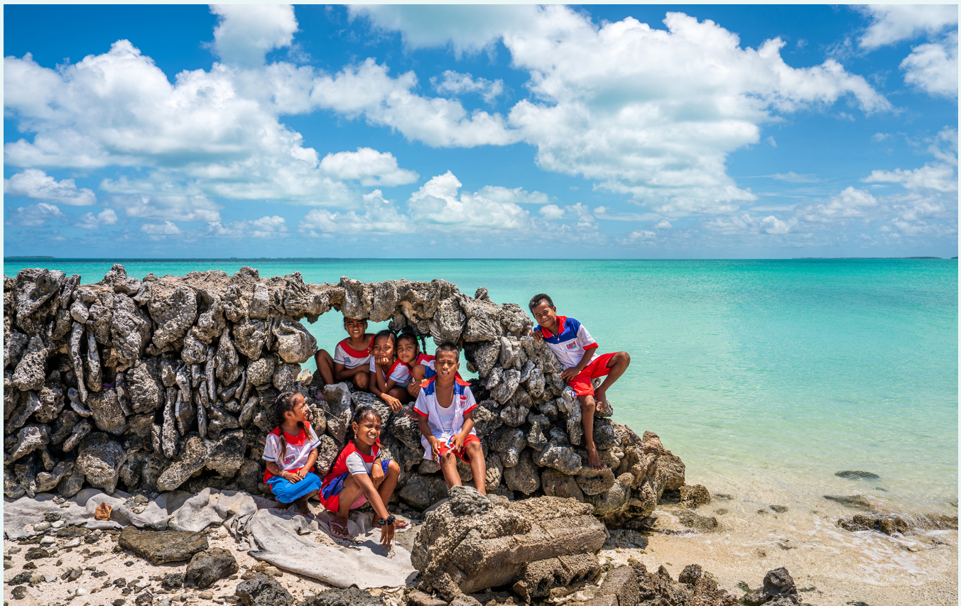
Children at a damaged sea wall in Tebunginako Village, which has been severely affected by rising sea levels, on Abaiang Island. Kiribati, 2023. | PHOTO UNICEF/FAUZAN
